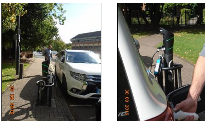
Figure 0.1 – Example of an Electric Charging Point
